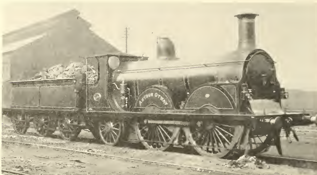
FIG. 343—W. STROUDLEY'S FOUR-COUPLED EXPRESS ENGINE. "GLADSTONE" CLASS. L.B. & S.C.R., 1882-91 (Photo. Locomotive)
