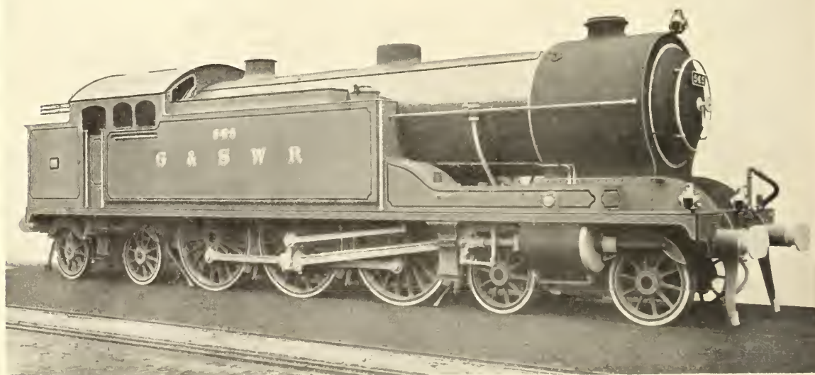
FIG. 473—R. H. WHITELEGG'S "BAL TIC" TYPE TANK ENGINE, GLASGOW & SOUTH-WESTERN RLY., 1922
