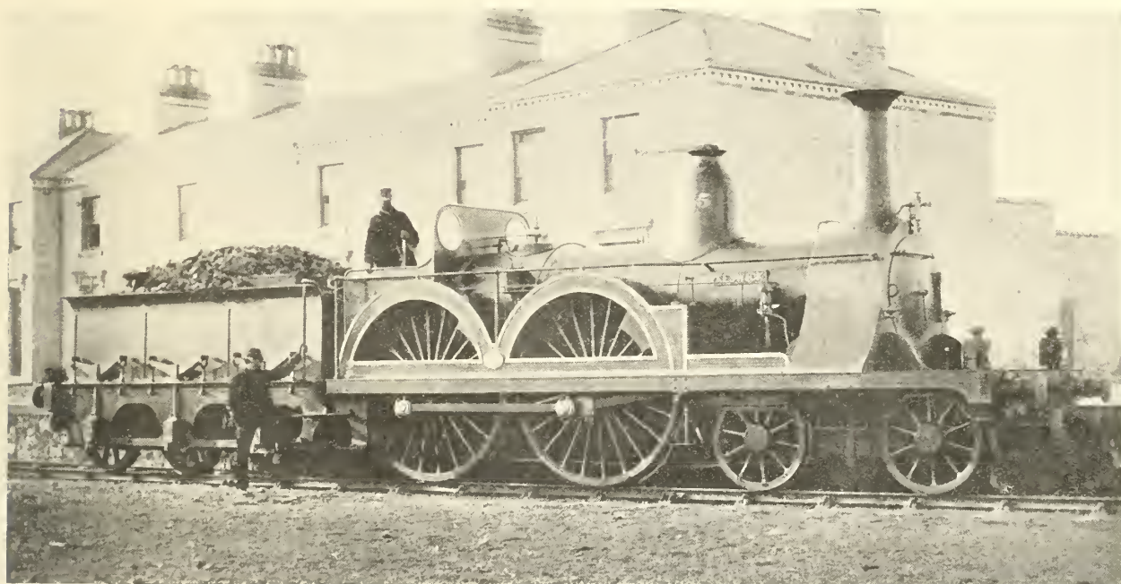
FIG. 187. STEPHENSON'S BOGIE PASSENGER ENGINE FOR THE STOCKTON & DARLINGTON RLY., 1862 [Photo. Locomotive]
