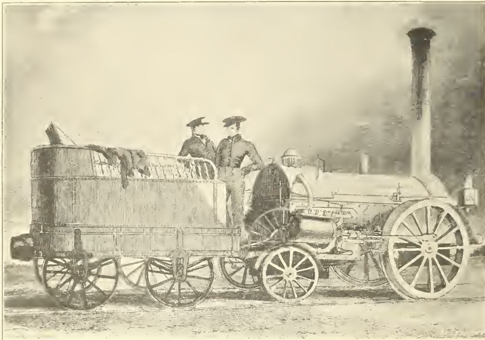
FIG. 9—THE "NORTHUMBRIAN," LIVERPOOL AND MANCHESTER RAILWAY, BY R. STEPHENSON AND CO., 1830
