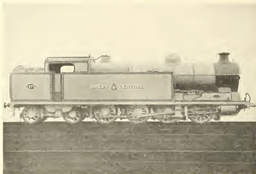
FIG. 426—J. G. ROBINSON'S THREE-CYLINDER SHUNTING ENGINE, GREAT CENTRAL RLY., 1907
