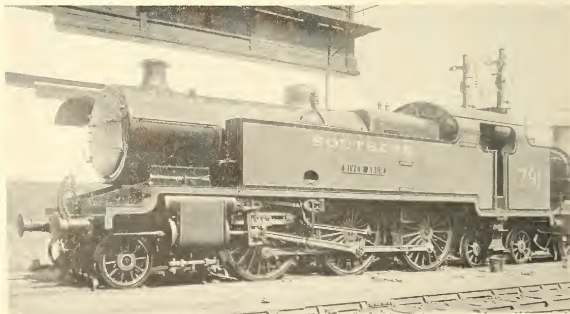
FIG. 465—R. E. L. MAUNSELL'S 2-6-4 PASSENGER TANK ENGINE, SOUTHERN RLY., 1917-25
