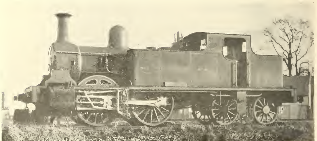
FIG. 292—SINGLE FAIRLIE TANK ENGINE, SWINDON, MARLBOROUGH & ANDOVER RAILWAY, 1878
